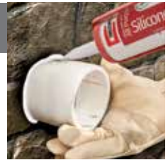
Caulk wall opening.
