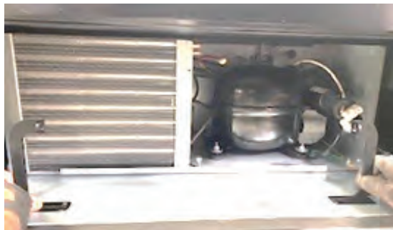
Figure 26 – Refrigeration deck removal
