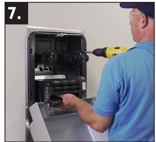
Attach dispenser to the wall studs using 4 screws through the screw bosses (Screws are not included with dispenser).
