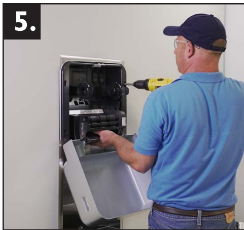
Drill mounting holes through the flange.
