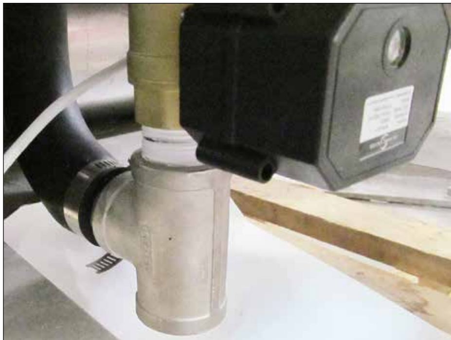
Fig. 7 - 1" NPT electric drain valve connection
