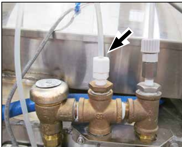
Fig. 20 - Rinse aid injection point
